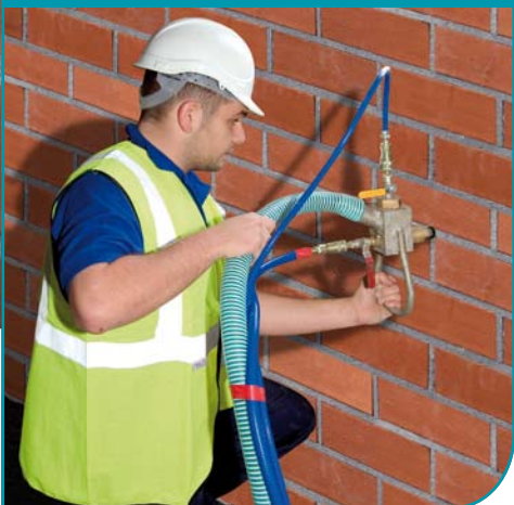
EcoBead installed externally
